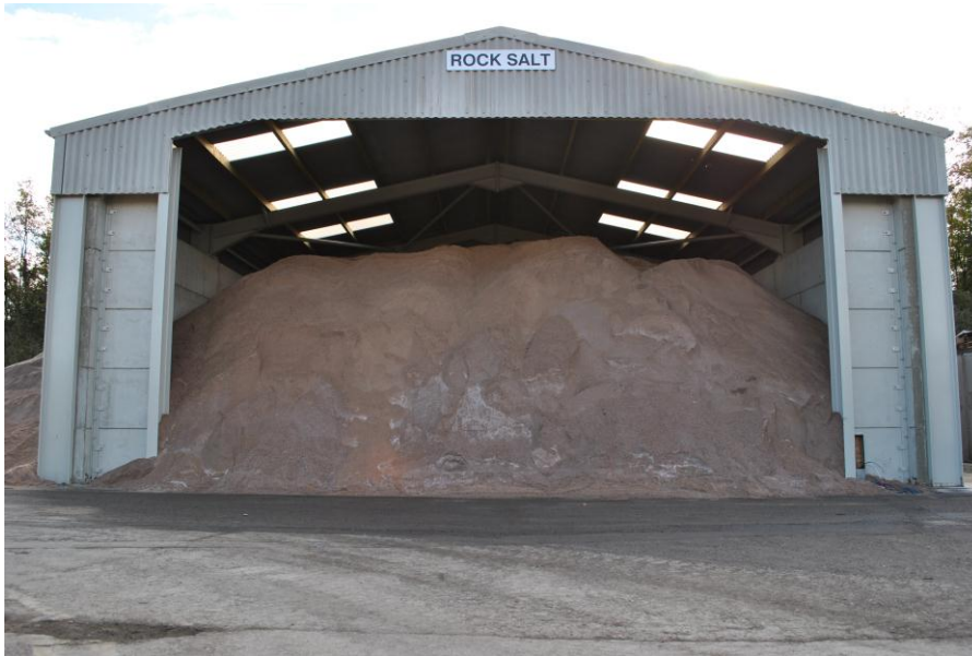
Salt barn Storage capacity 850t
